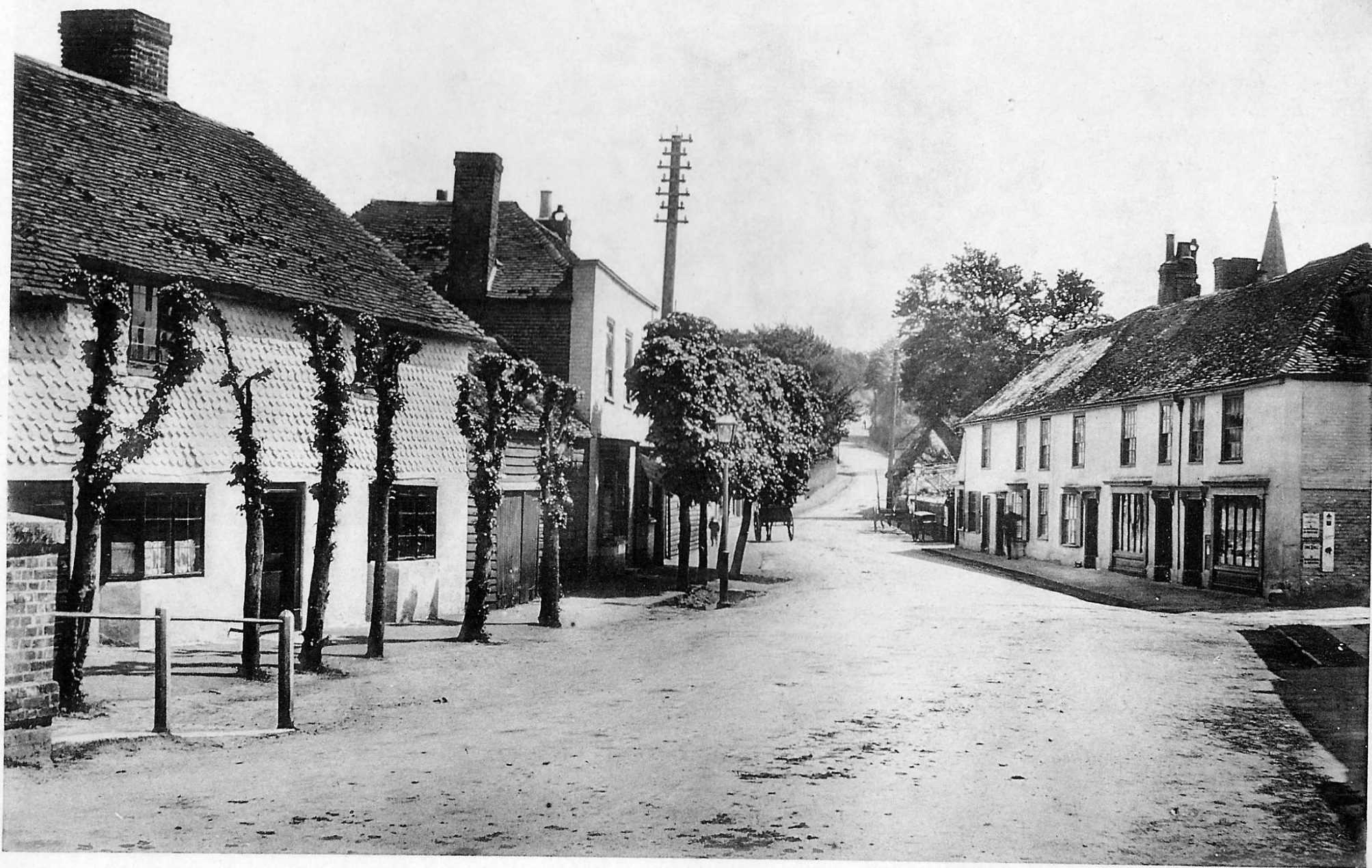
Bridge Hill from High Street.
