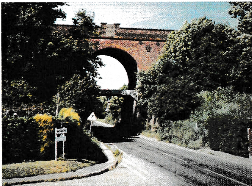
The Railway Bridge
