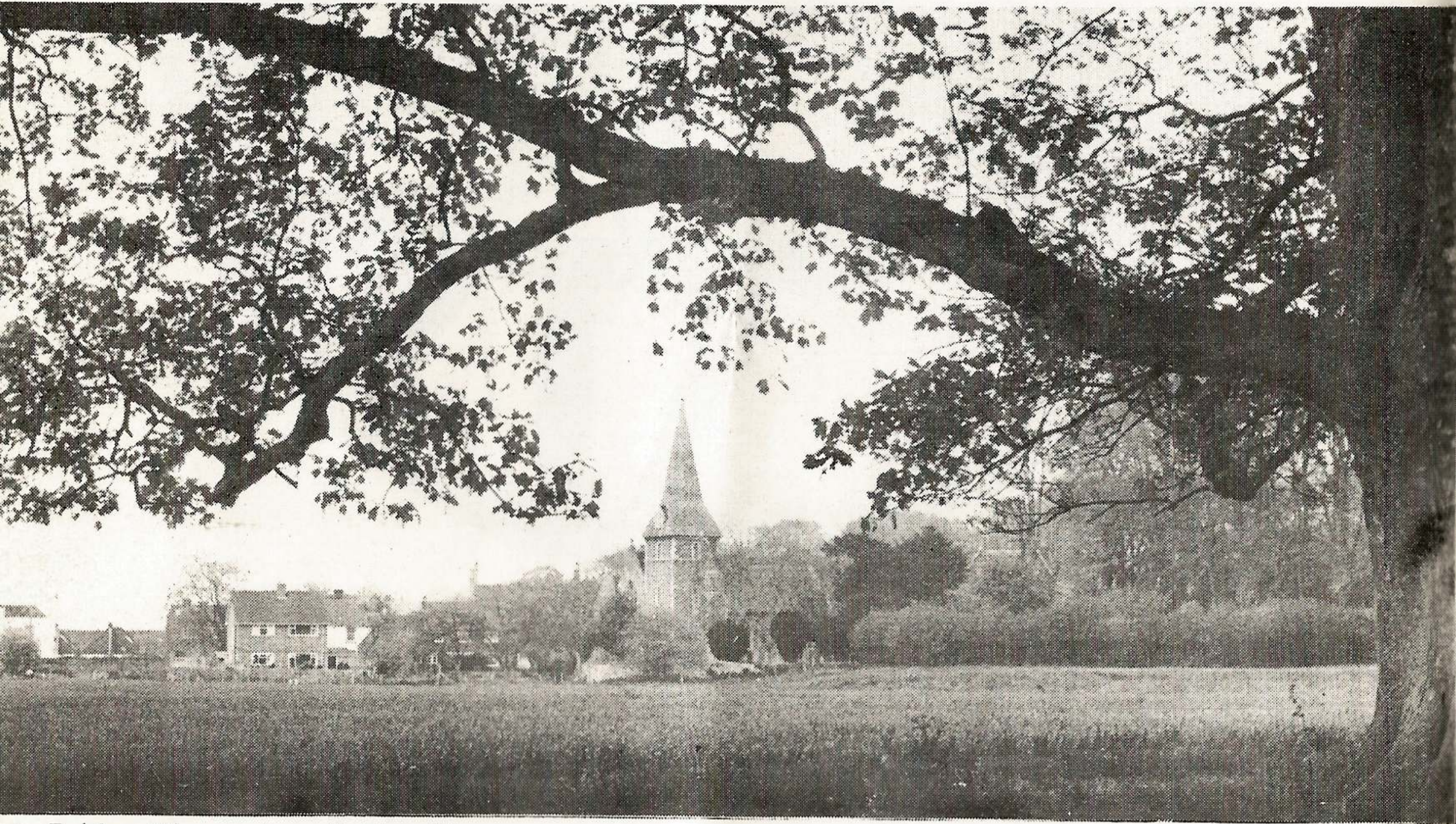
Bridge Church from Bridge Place.
