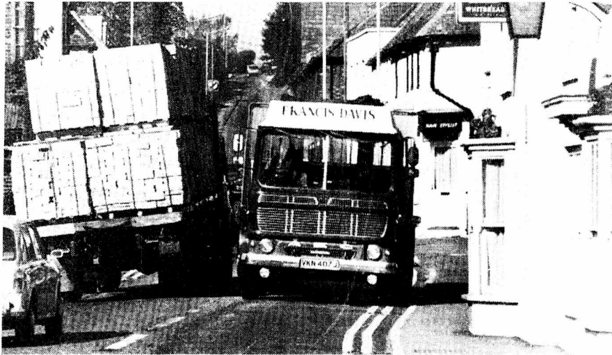
a picture of Bridge we are happy to lose; heavy traffic the High Street in 1972. Picture courtesy of the Sunday
