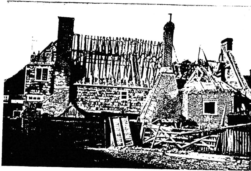
A. View of rear of the house.
