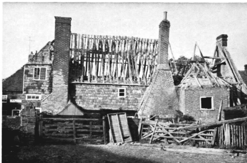
A. View of rear of the house.
