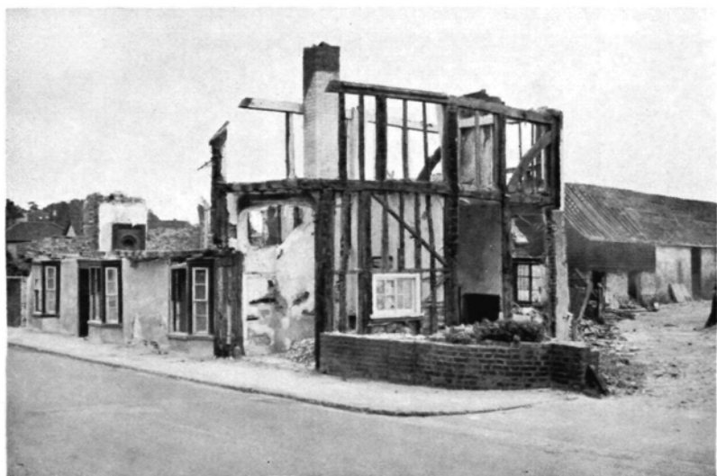
B. Same view later, showing wagon entrance.
