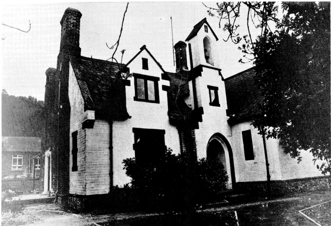
Bridge and Patrixbourne School, constructed in 1849, as it appears in 1978.
