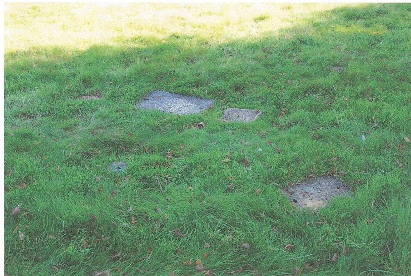
Fig. 9. Iron utility covers.
