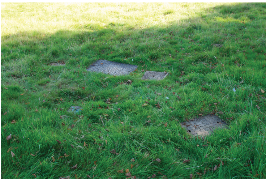
Fig. 9. Iron utility covers.
