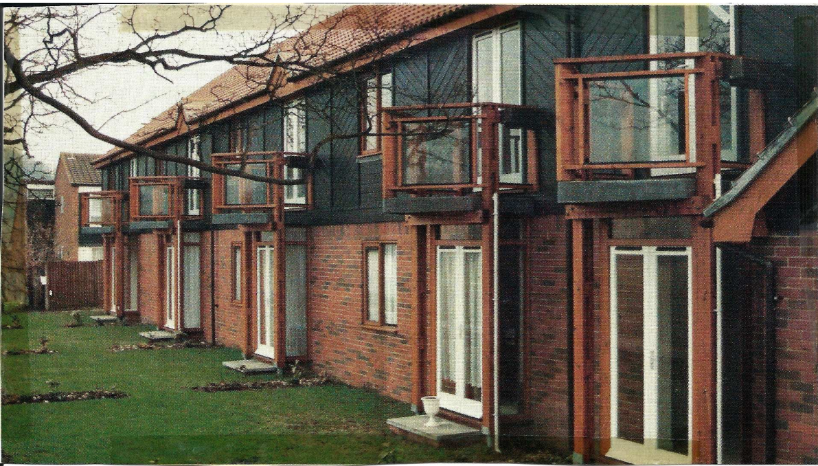
2 Riverside Close, Bridge, Nr. Canterbury. A sheltered housing scheme for Ansley Abbott (Homes) Ltd., balcony detail.
