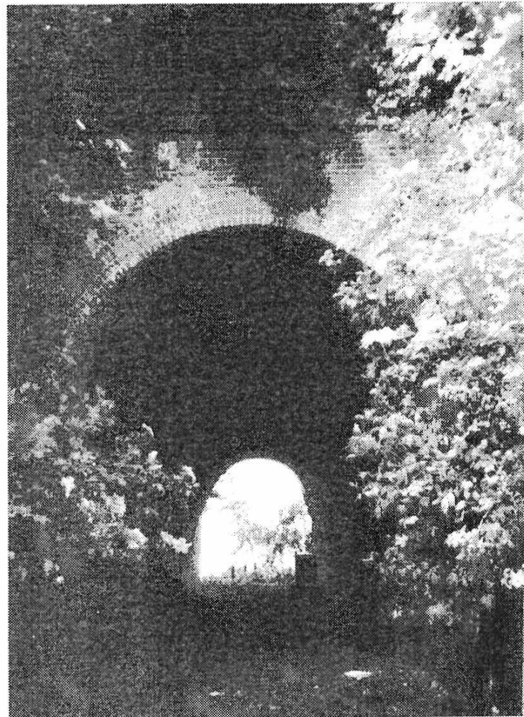
5 The Tunnel or "Long Arch"
