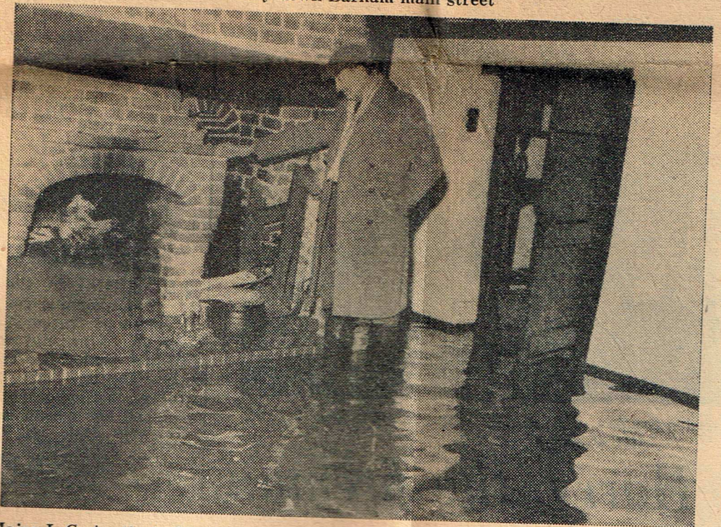
Major I. C. Austin in his flooded Barham home . . . the water rose through the floor, sweeping away the parquet flooring
