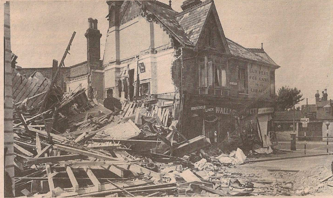
This building in Rock Avenue, Gillingham was destroyed during a raid
