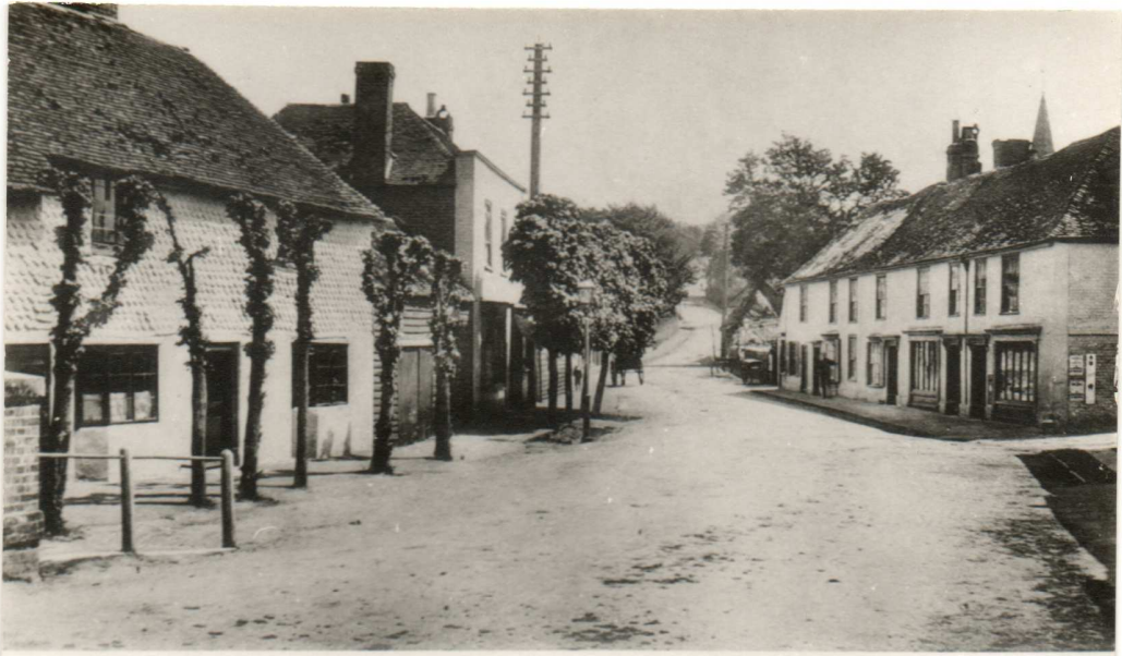
Bridge Hill from High Street.
