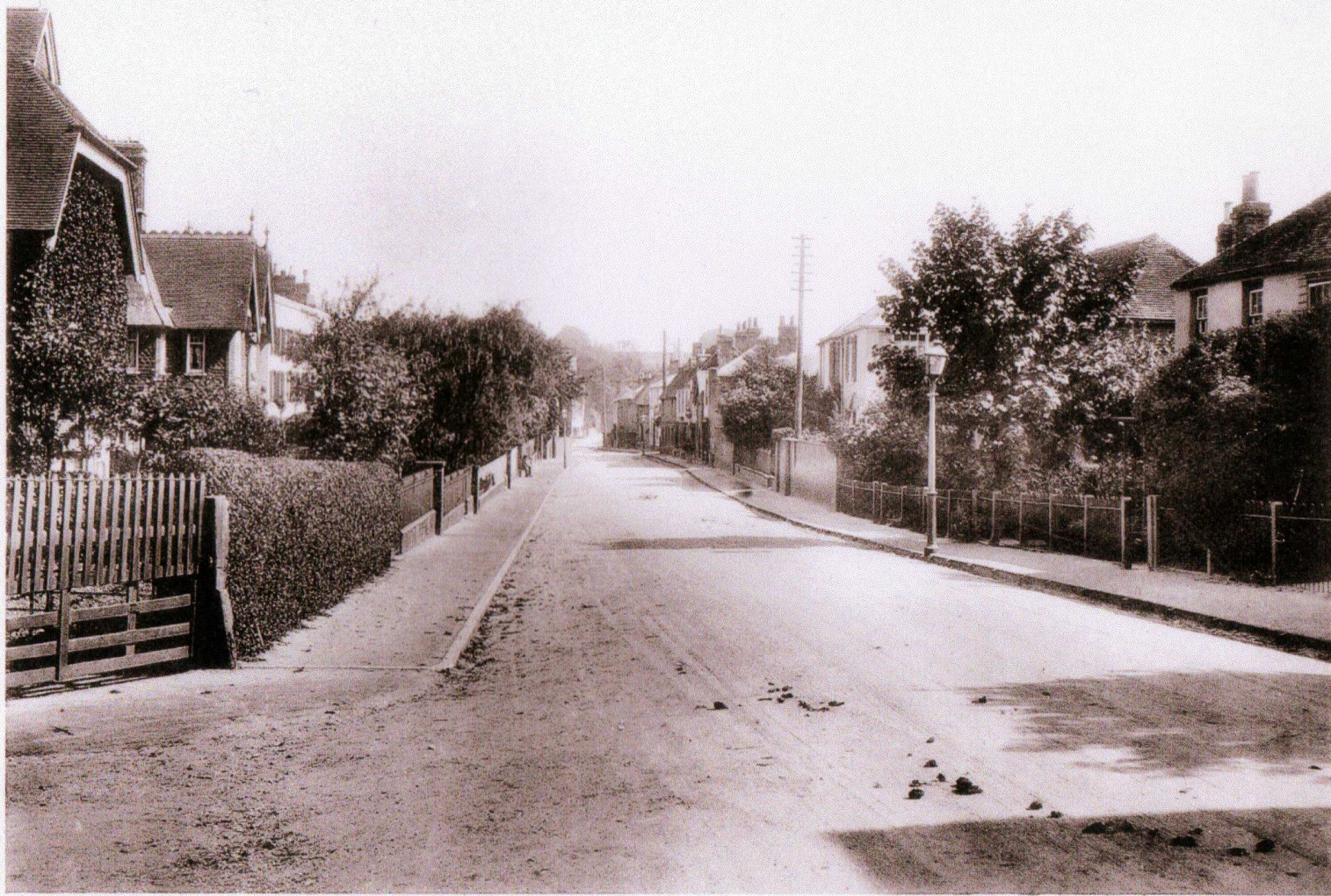
Bridge, from Canterbury Hill.
