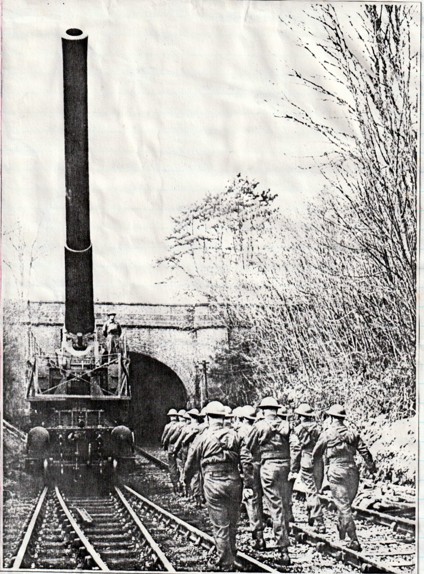
Drill session in progress outside Bourne Park tunnel with 'Boche Buster' menacingly pointing skywards.
