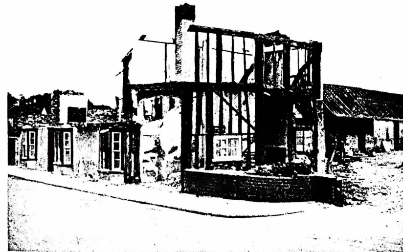
B. Same view later, showing wagon entrance.
