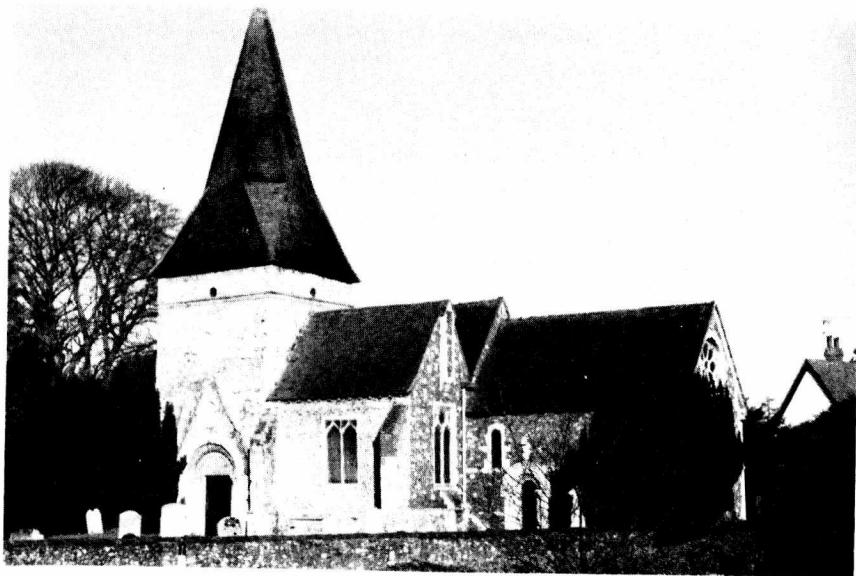
Patrixbourne church, showing the tower with the south doorway beneath, the chancel and the narrow south aisle.
