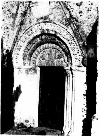
The decorative Norman doorway of Patrixbourne church, showing the triangular canopy enclosing an arch niche.
