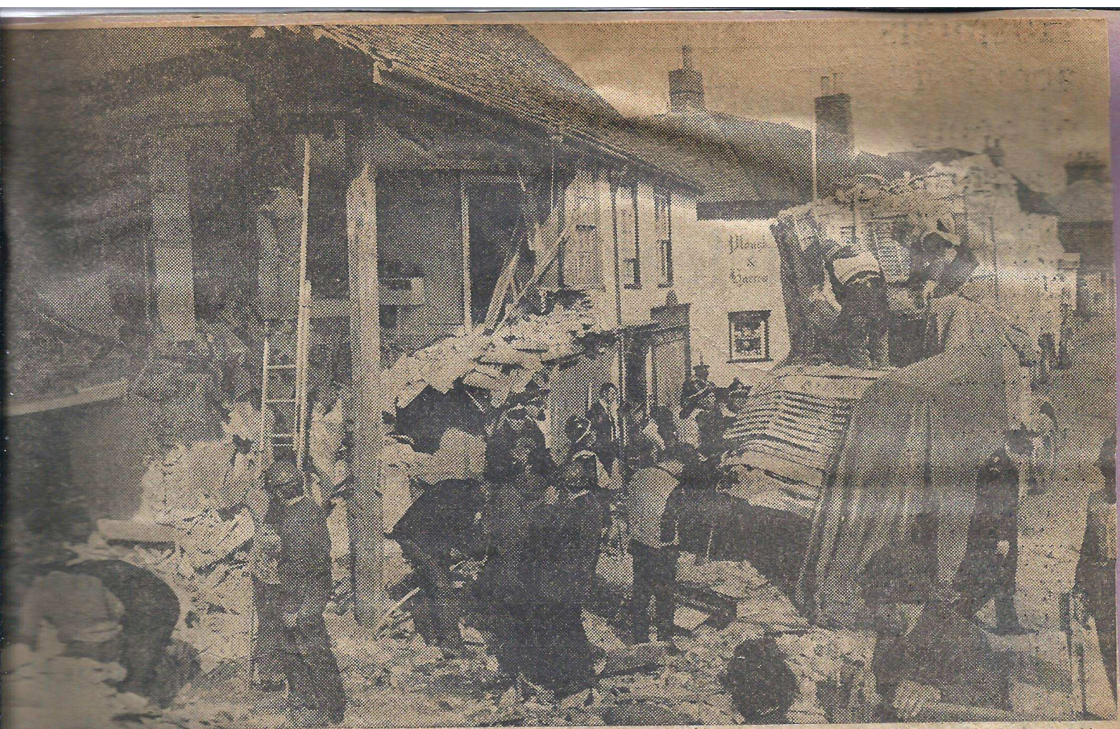
Rescue workers and other rescue workers in Bridge, near Canterbury, yesterday, after a 30-ton lorry had crashed into a row of shops. It took six hours to release the body of the driver, Mr Reginald Christopher, aged 53, of Dagenham. Angela Lewis, aged 15, daughter of village grocer, was flung across her bedroom by the impact.
