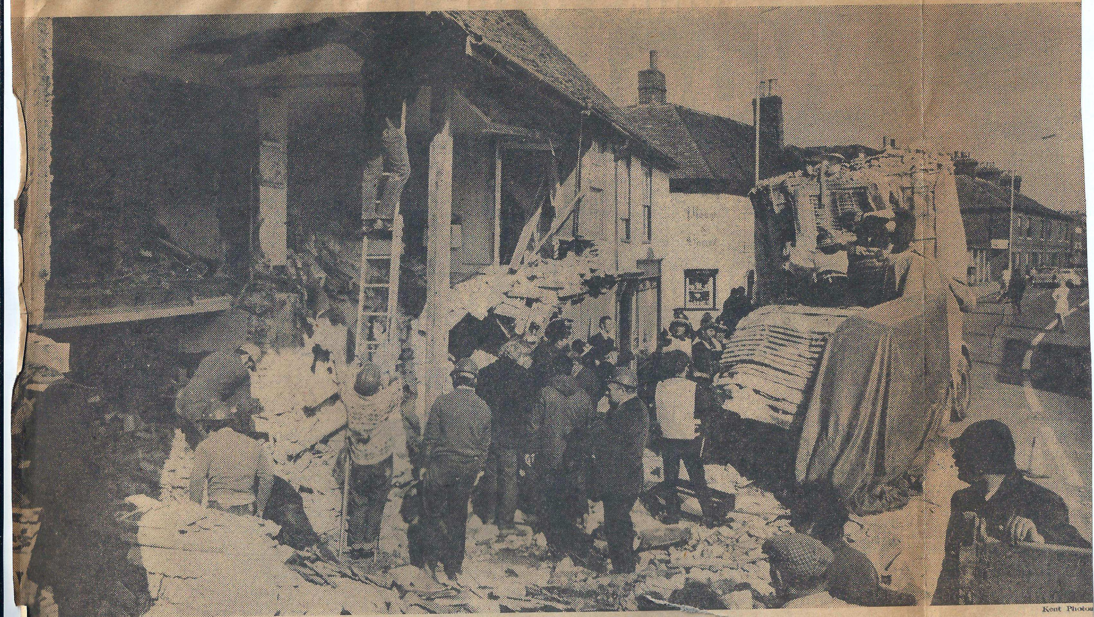
THE SHOP—This was the scene in Bridge village main street after the crash today.
