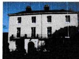
(23) East Bridge House
