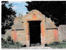
(47) Doorway to 'Hillside' 57
