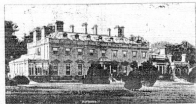
A view of the south front of Bifrons, c. 1700.
