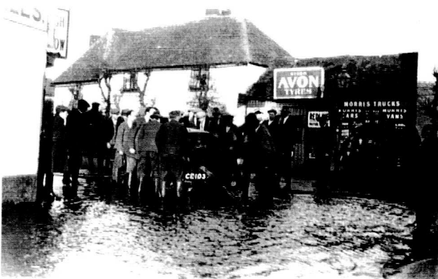
Fire Brigade pumping out flood
