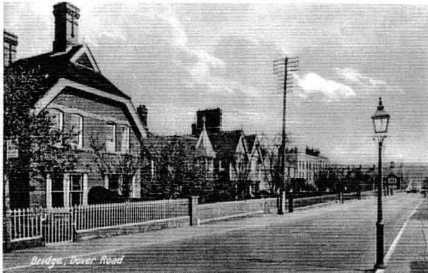
Bridge, Over Road
