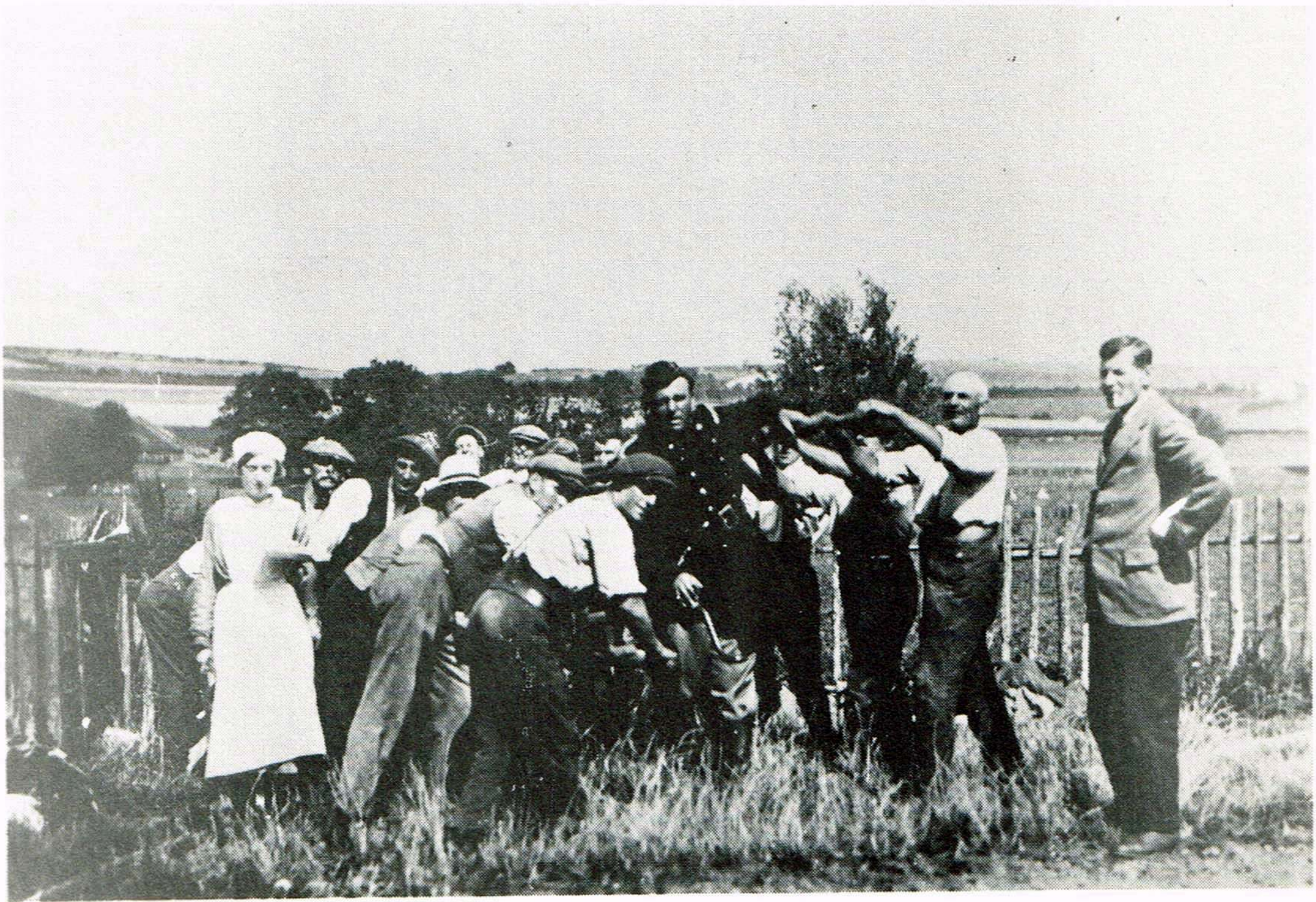
Bridge Volunteer Fire Brigade testing Merryweather Hand Pump in case of fire.
