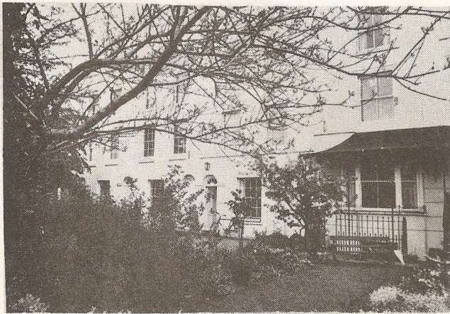
Albany Terrace, The High Street, Bridge.
