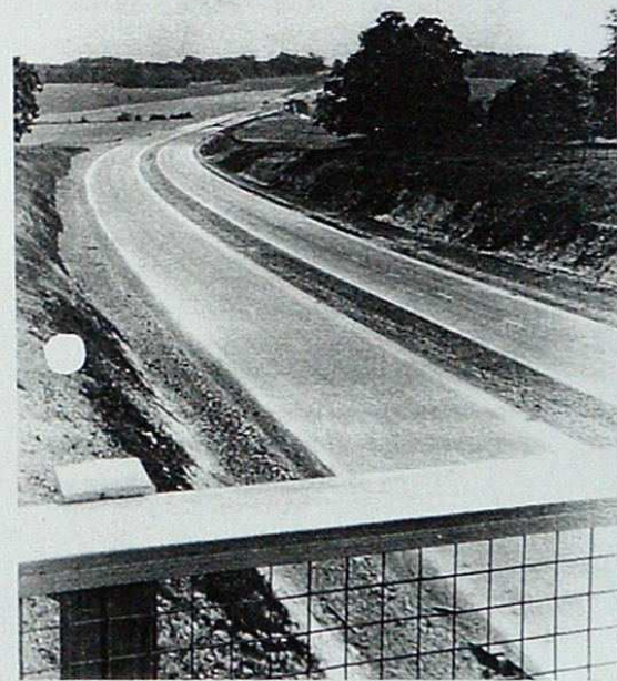
Looking towards Dover from Bekesbourne Bridge.
