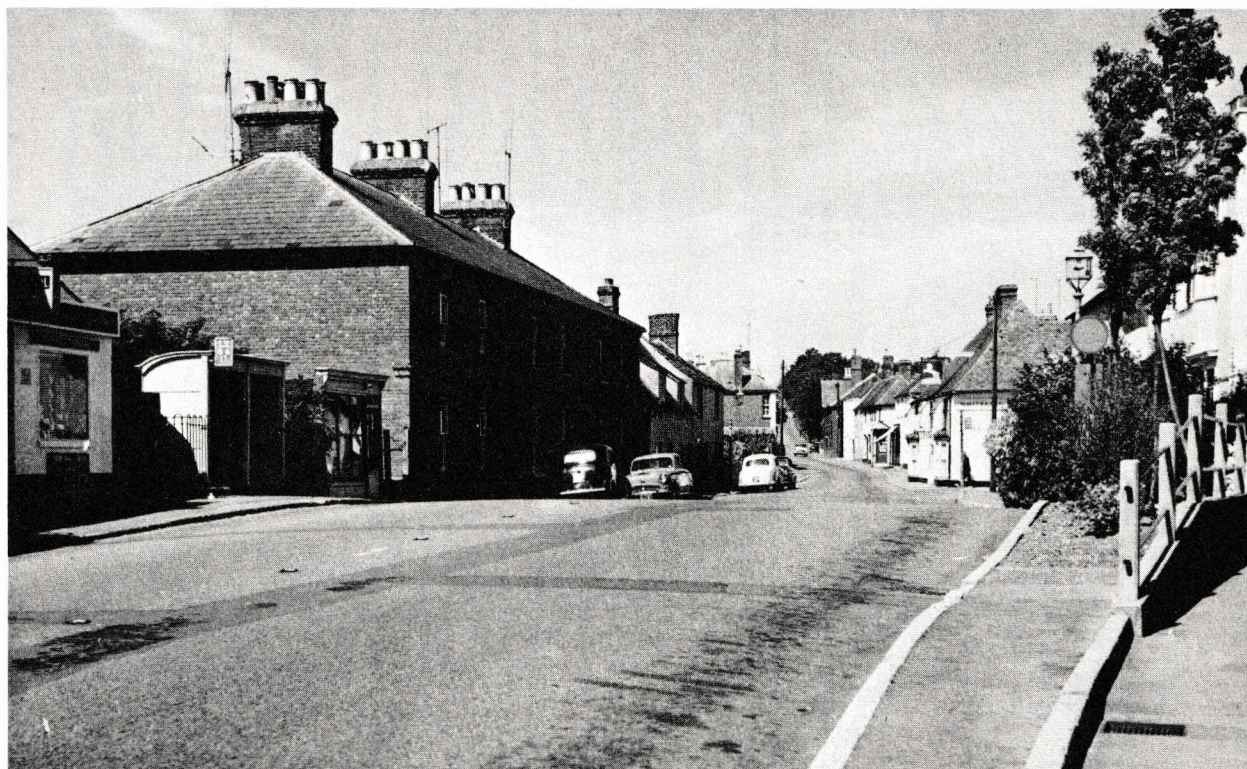
High street Bridge Kent looking north. From a photograph by Brian Pearson taken in the early 1960s. (See note on page 44)
