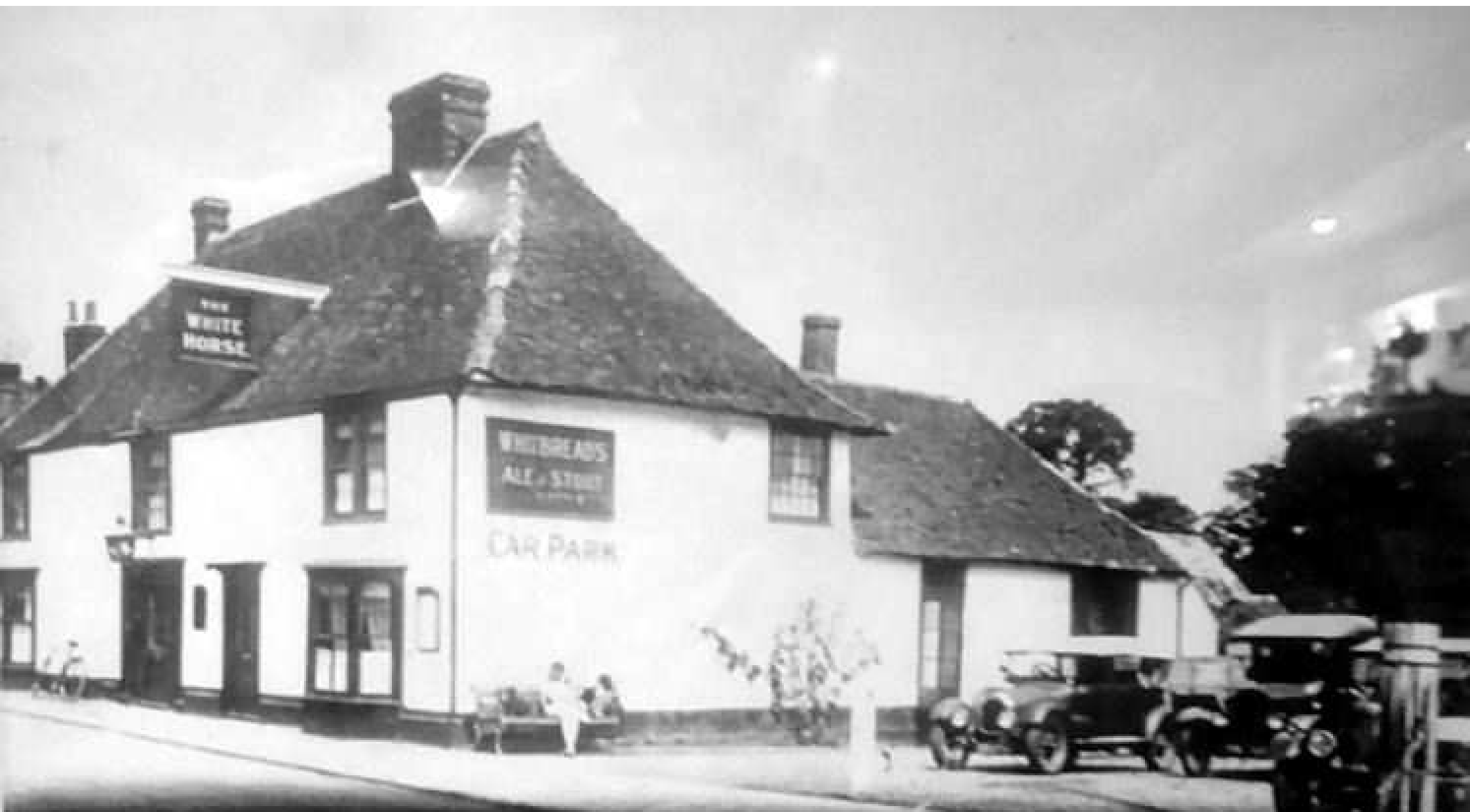
"THE WHITE HORSE", BRIDGE, NEAR CANTERBURY KENT. (Phone: BRIDGE 49.) Proprietor, W. J. FAIRSERVICE. (KENT COUNTY CRICKET XI. 1902-1921). FULLY LICENSED.
