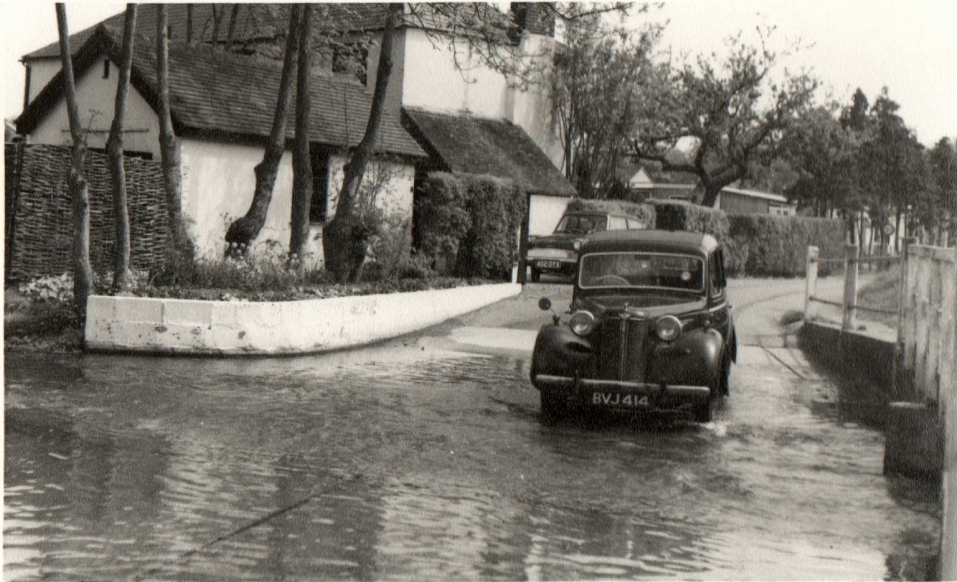
Bridge, Kent, A Real Photograph. J.M.
