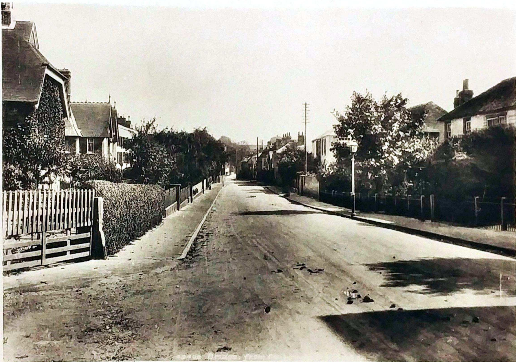
Bridge, from Canterbury Hill.
