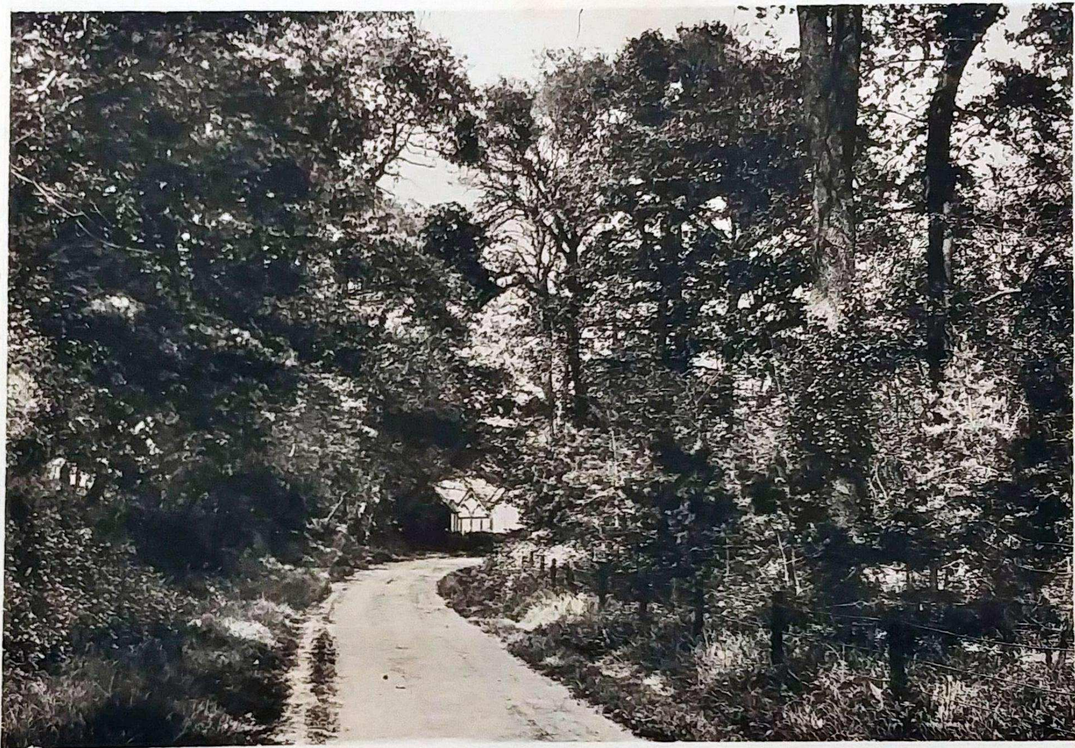
Bridge, Laundry Lane.
