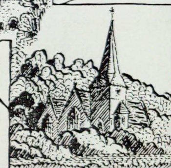
ST PETER BRIDGE
