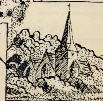
St PETER BRIDGE
