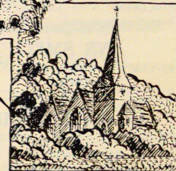
ST PETER BRIDGE
