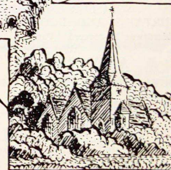
St PETER BRIDGE
