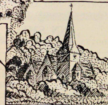
ST PETER BRIDGE
