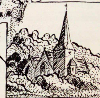
St PETER BRIDGE
