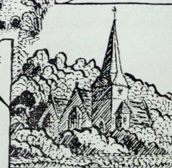
ST PETER BRIDGE
