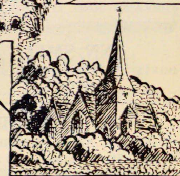
St PETER BRIDGE
