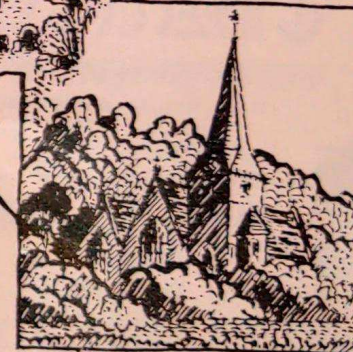
ST PETER BRIDGE
