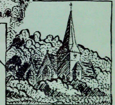
St PETER BRIDGE
