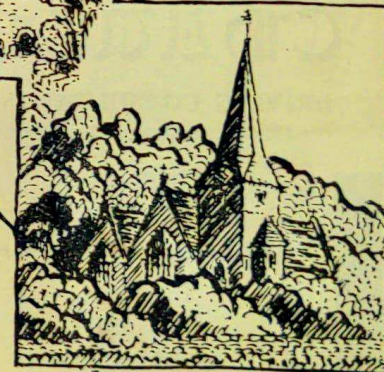
St PETER BRIDGE
