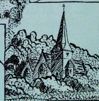
ST PETER BRIDGE
