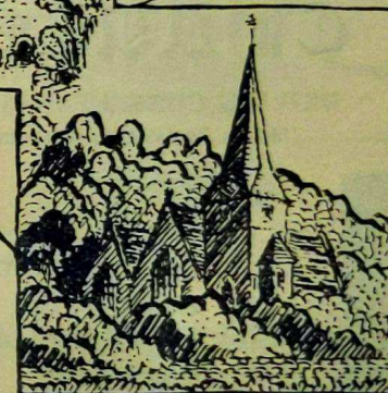
St PETER BRIDGE
