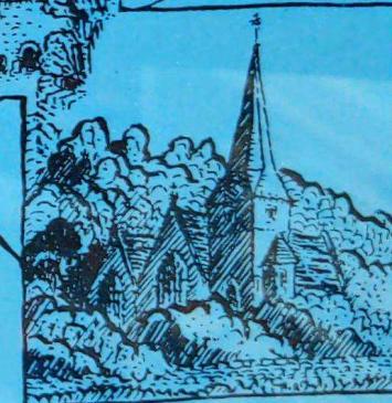
ST PETER BRIDGE
