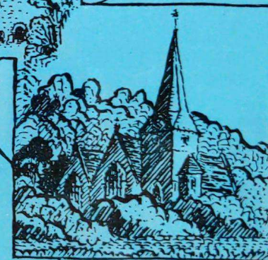
ST PETER BRIDGE
