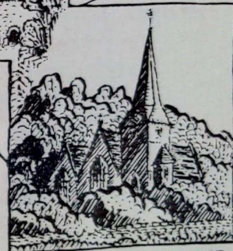
St PETER BRIDGE
