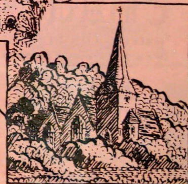
St PETER BRIDGE
