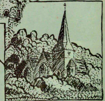
St PETER BRIDGE
