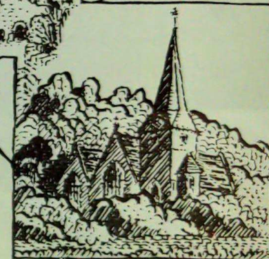
St PETER BRIDGE
