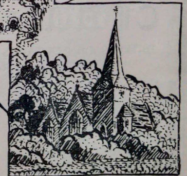
St PETER BRIDGE
