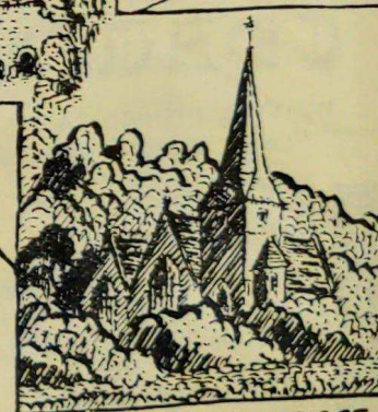
St PETER BRIDGE
