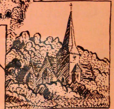
St PETER BRIDGE
