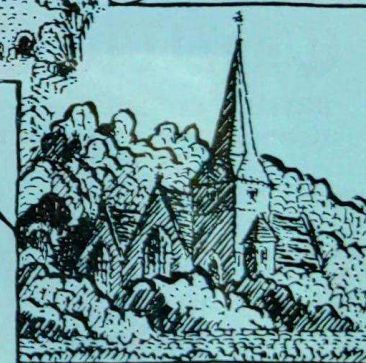
St PETER BRIDGE
