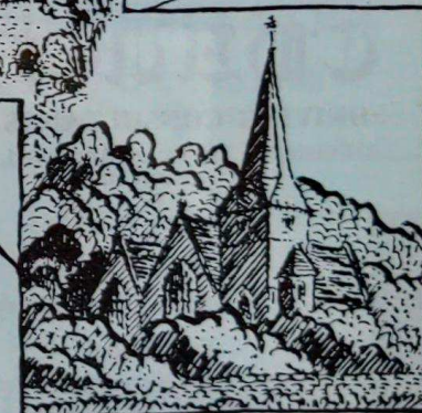
St PETER BRIDGE
