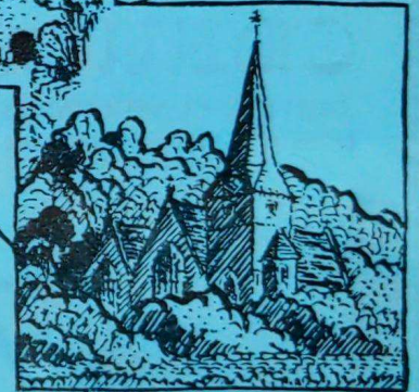
St PETER BRIDGE
