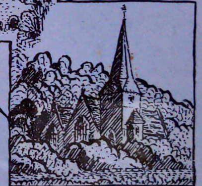
St PETER BRIDGE
