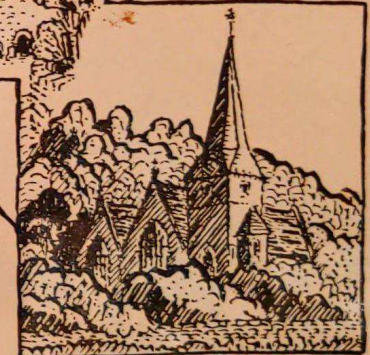
St PETER BRIDGE
