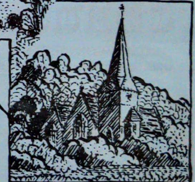
St PETER BRIDGE
