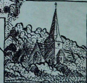
St PETER BRIDGE
