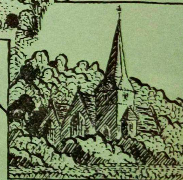
St PETER BRIDGE
