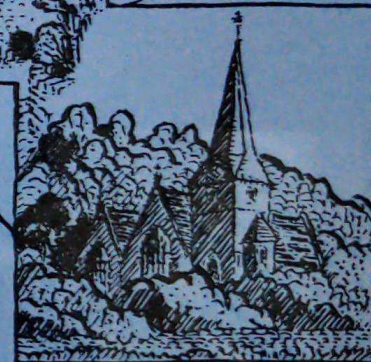
St PETER BRIDGE
