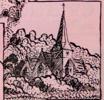
St PETER BRIDGE
