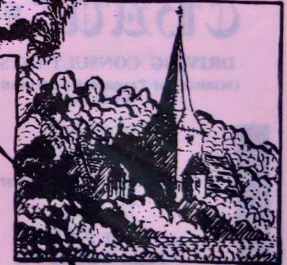
St PETER BRIDGE
