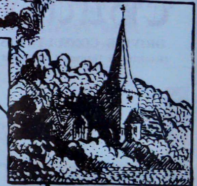
St PETER BRIDGE
