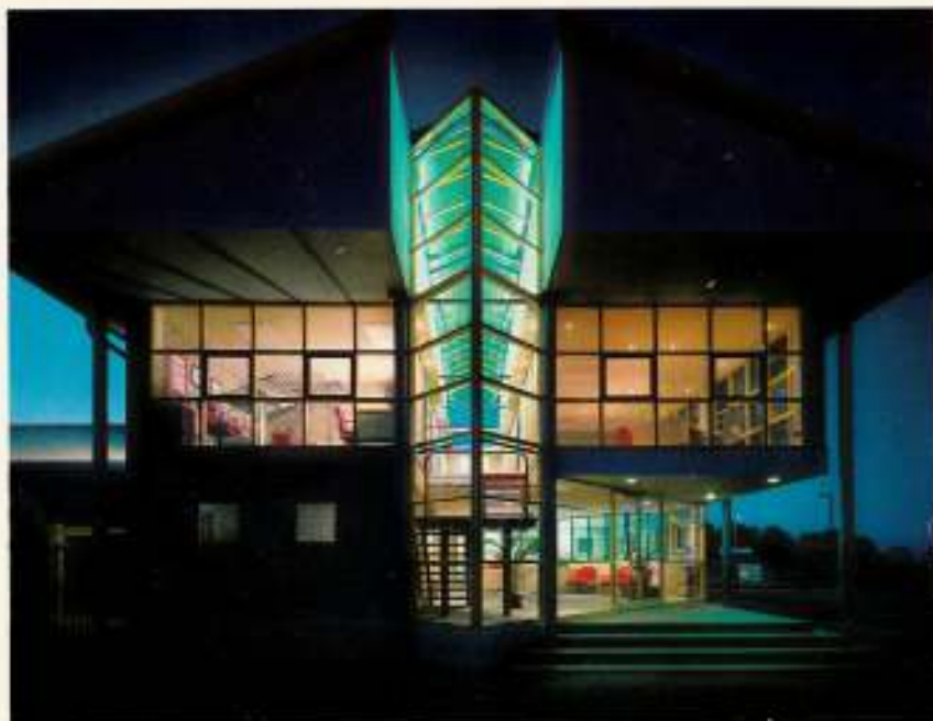
Head Office - Knight Builders (Canterbury) Ltd.
