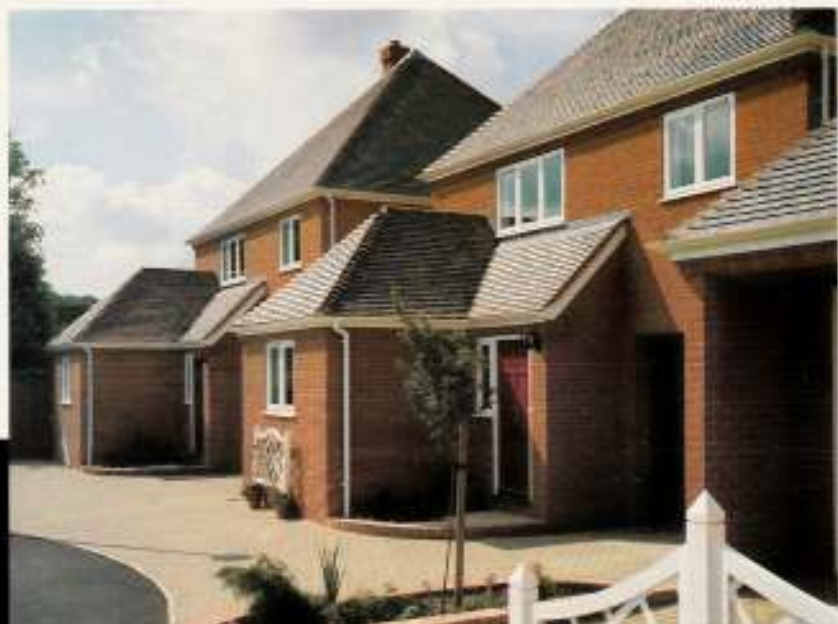
Design & Build Development, Bridge.
