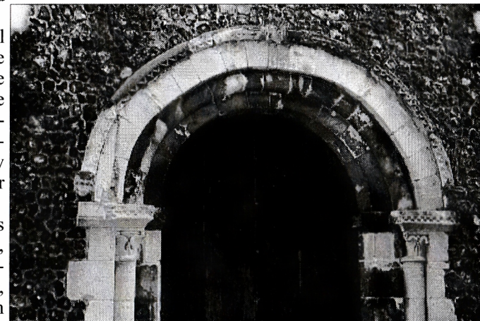
West window, top. West doorway, above.
