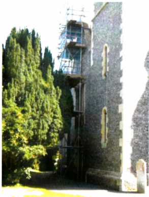
Scaffolding bracing the West wall
