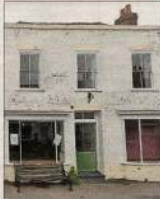
The redundant site in Bridge high street
