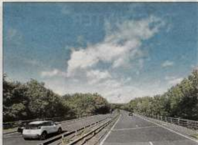
The A2 will have lanes narrowed and speed restrictions as well as overnight closures during the works
