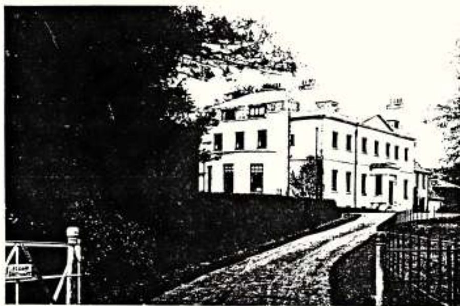
Higham House (left driveway)
