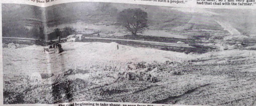
The road beginning to take shape, as seen from Bifrons Park in February, 1975.
