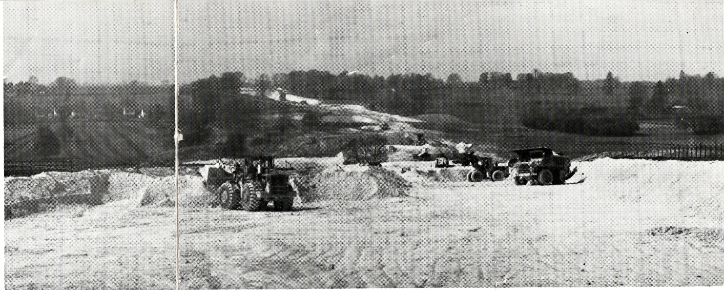
The line of the bypass is becoming apparent as teams of excavators and lorries move chalk in April 1975.
