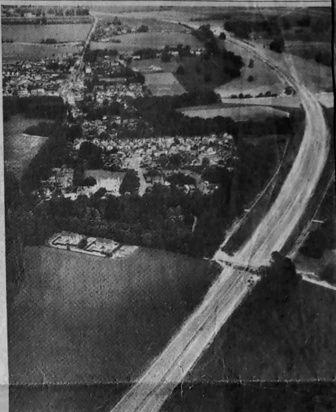
A bird's eye view of Bridge's £3½ million by-pass which opened after a 14-year campaign on Tuesday. The dual carriageway road, completed two months ahead of schedule, will mean a return to the old, peaceful way of life for villagers.
