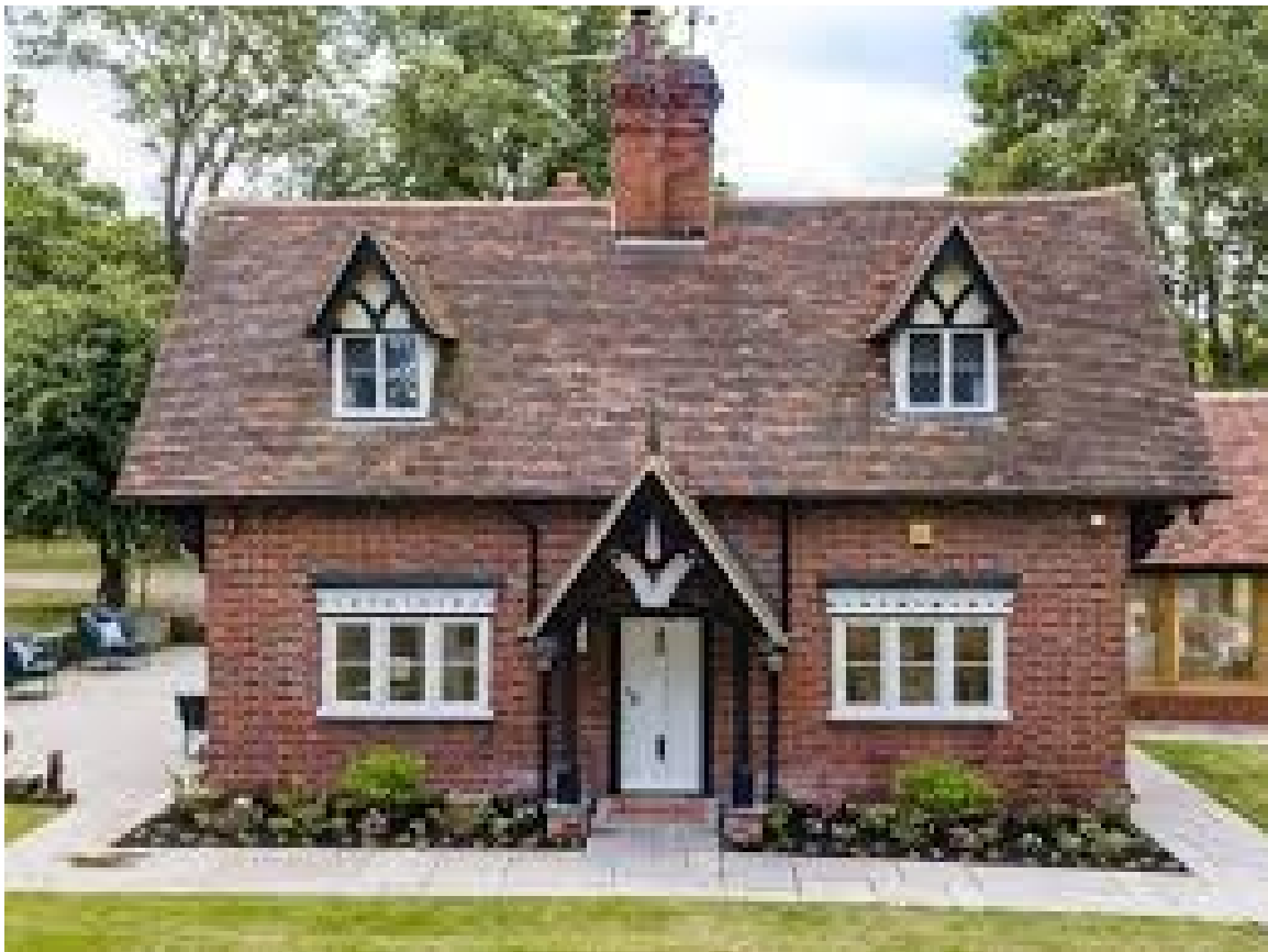
Keeper's Cottage once the home of keeper Poland
